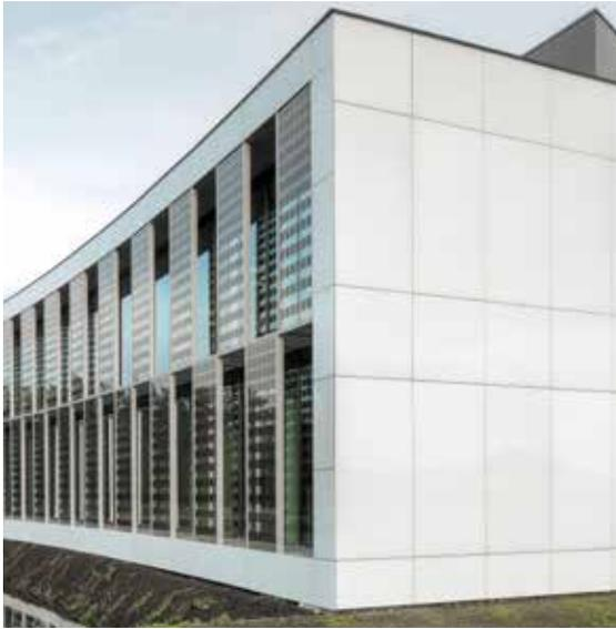
**Projects:** to ensure a uniform appearance and color across a given project, AGC recommends using Lacobel T and Matelac T glass made from a **single production batch, heat treated on the same furnace, helping to ensure a uniform direction of roller-wave throughout the project** (from cutting to installation).
